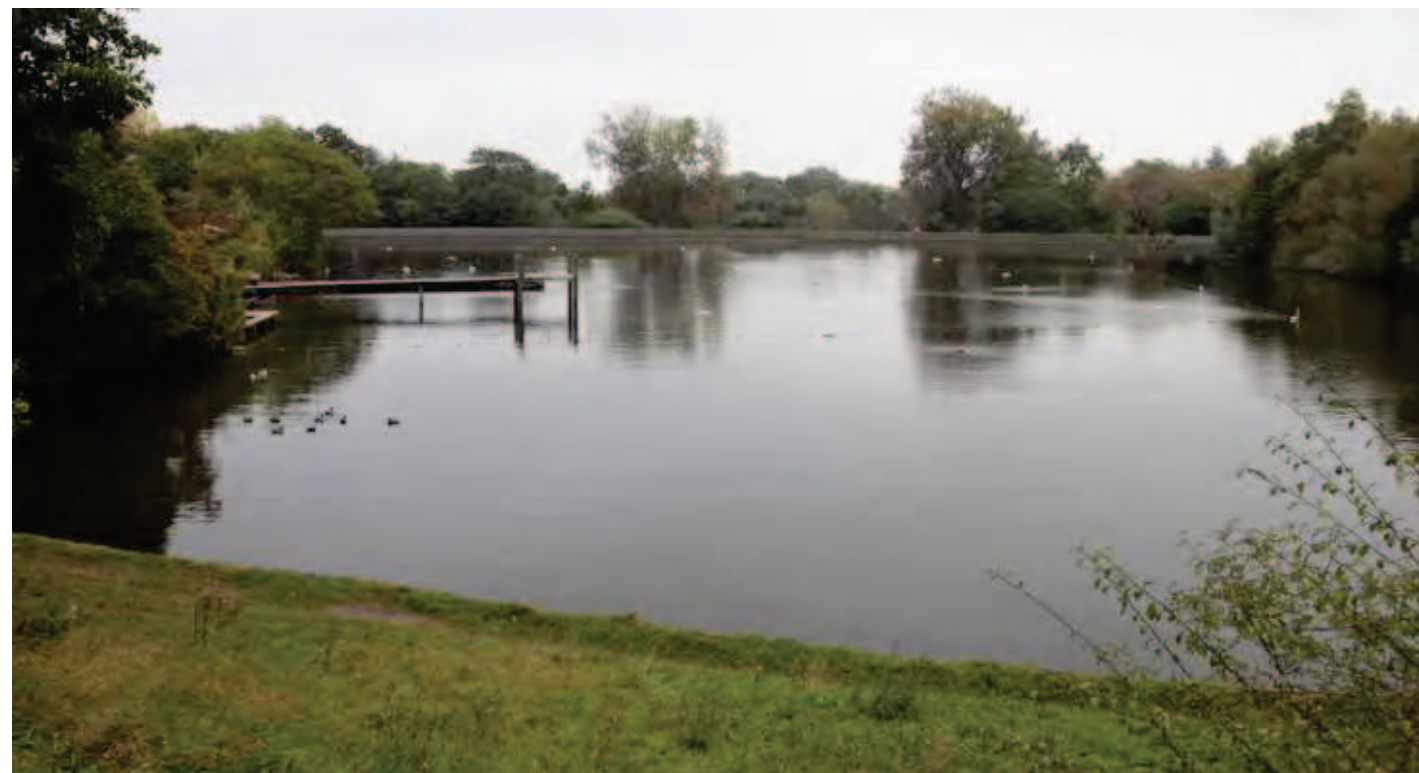
View Point 9 - View across Mens Bathing Pond looking South , showing one possible location of spillway 1.5m wall (Option 4)
