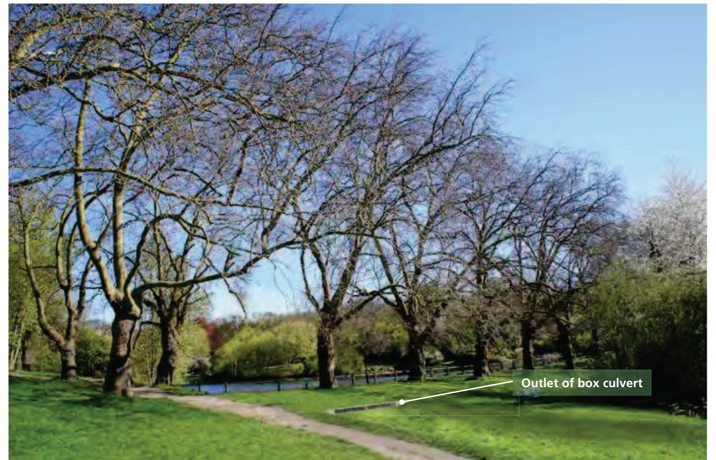
View Point 3 – North across Hampstead No. 2 Pond Box Culvert Spillway - 1 Plane Trees Lost, 400x5000mm culvert (Option P)
